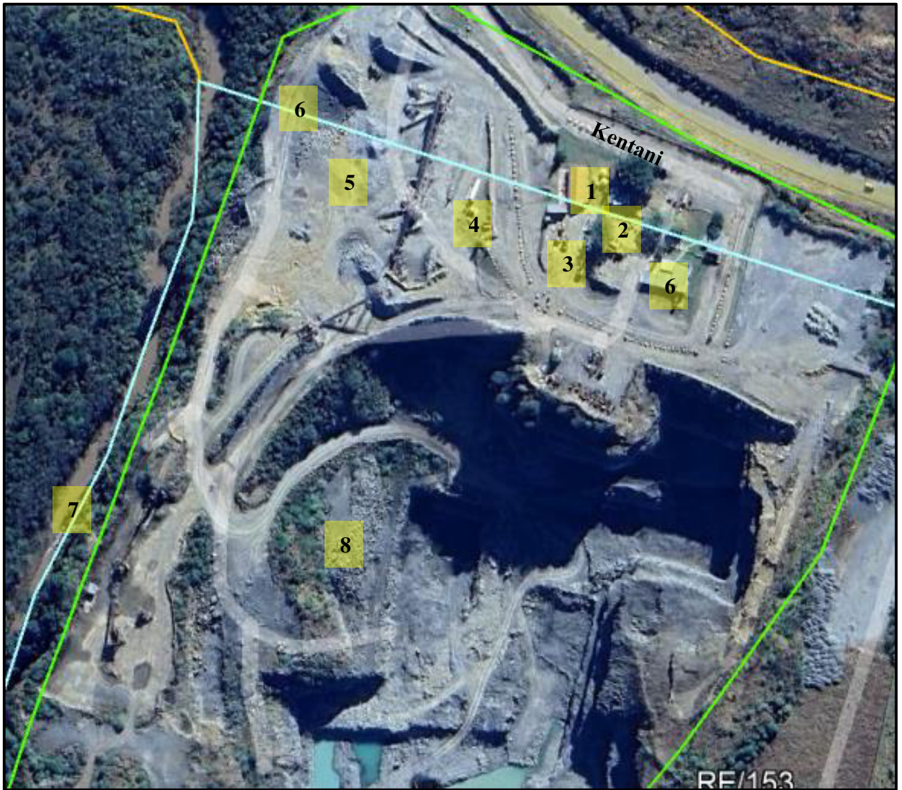
Figure 3: Satellite view of the various developed areas at Butterworth Quarry (image obtained from Google Earth)
